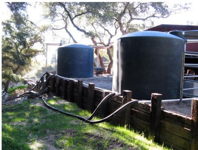
*This rain catchment system collects water from roof and gutters and stores it for future use or for slow release after the storm.*
