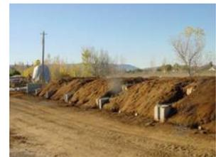
**The Free-Standing Aerated Static Pile and Block Bays** are well suited to flat ground conditions. The aerated static pile is the simplest and least expensive composting method. No structure is required; but block bays can be constructed, if desired. This approach simply includes pipes on grade attached to an aeration manifold or cast-in-place trenches to distribute the airflow evenly across the base of the pile.
