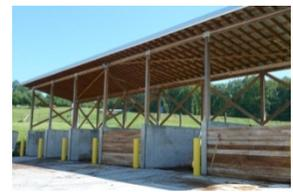
**The On-Grade Compost System** is perfect for farms and stables with flat topography. On-Grade systems have three or four bins, each with an aeration floor. They are designed to be constructed with lumber, although masonry block and concrete construction can also be used. Roof designs are included.
